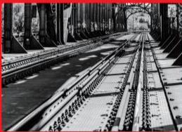
Road and bridge construction
