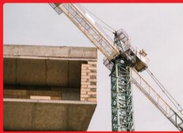
Large tower crane installation
