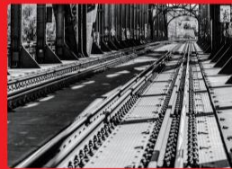
Road and bridge construction
